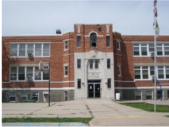
Pilger High School as it appeared in 2012, before the tornado hit the town.
