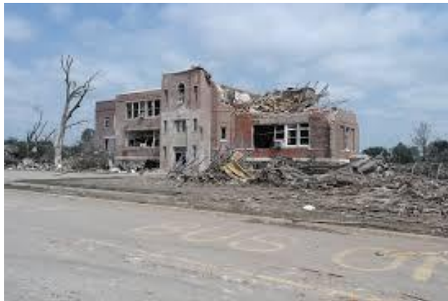
Pilger High School as it appeared after the tornado. The structure has since been torn down. The elementary students were moved to Wisner, a town just seven miles away.
