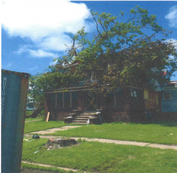
A tree comes to rest on the roof of a house
