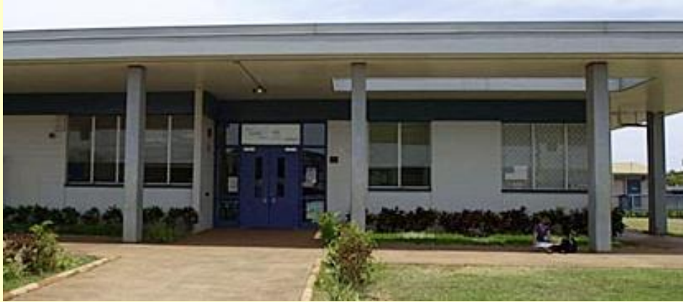
Administration building at Honowai Elementary School, Waipahu.
