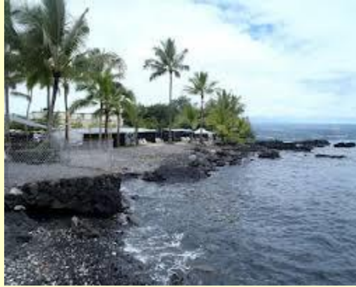
Main building at Richardson Ocean Center
