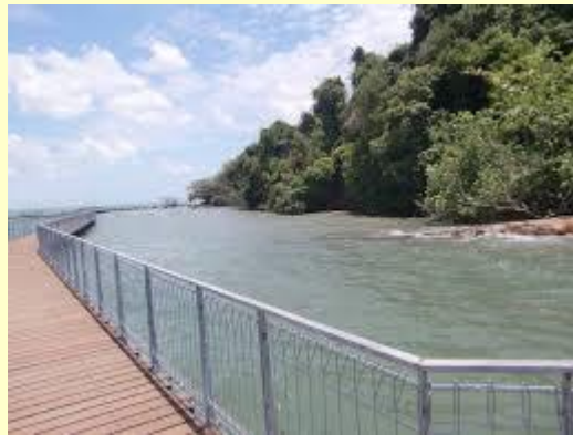
Chek Jawa Pulau Ubin walkway as it appears today.
