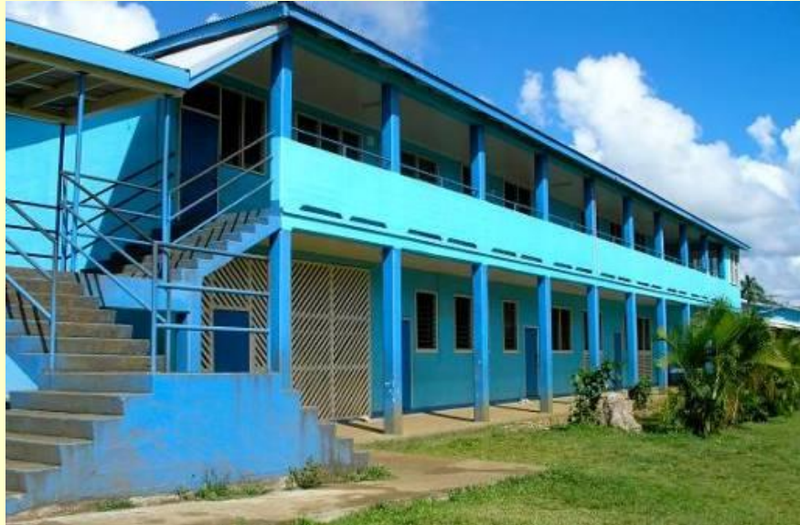
The main building of the Teachers Training College of Western Samoa in Apia
