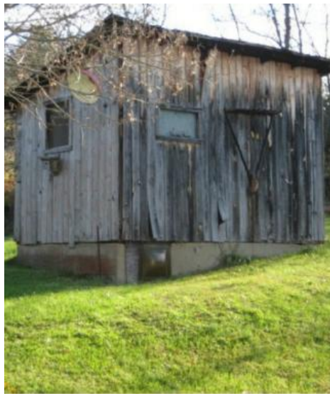
Old well house
