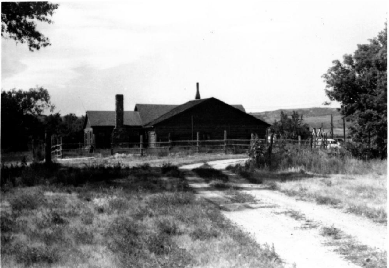
Jacobsen ranch house near Glendo, Wyoming
